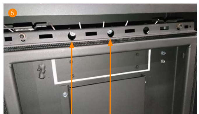
Holes for accessibility to measurement points
